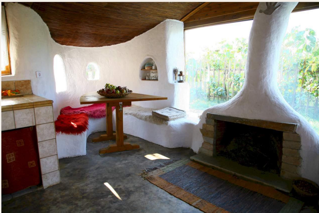
House and some furniture built in COB.
