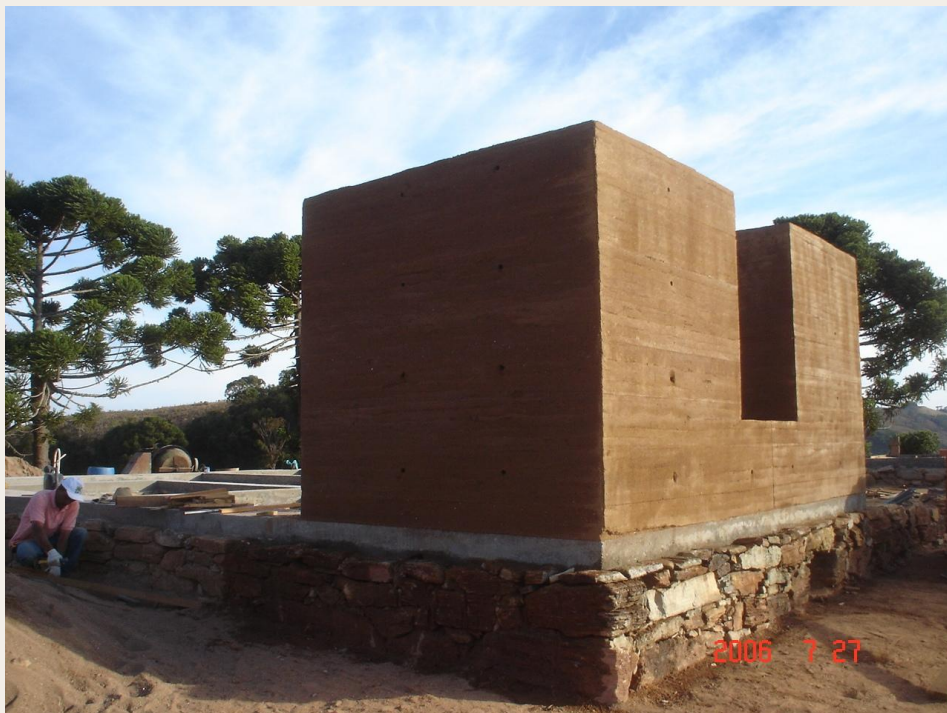
Rammed earth walls.
