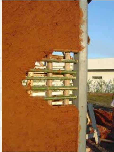
Detail of wall built with rammed earth by hando (bambboo-to-daub).
