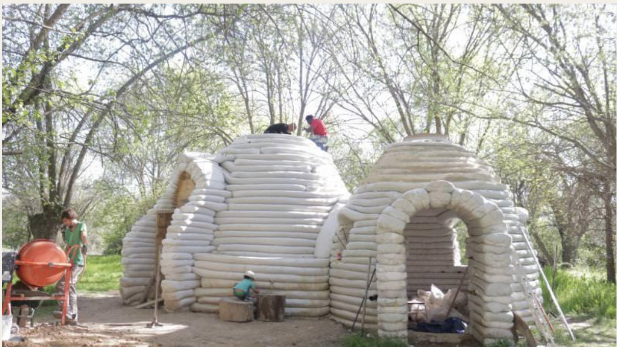
Construction in superadobe.
